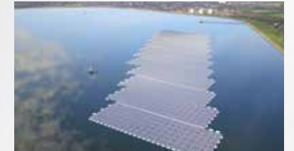
QE2, UK - 6,338 kWp
