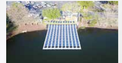
ORLANDO UTILITIES, USA - 32 kWp
