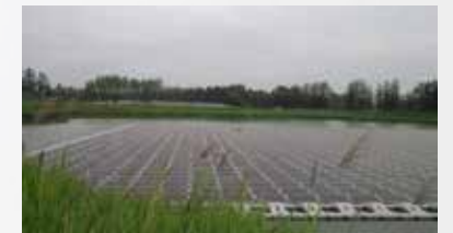
HEZE CITY, CHINA - 600 kWp
