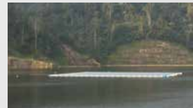
ULU SEPRI, MALAYSIA - 270 kWp
