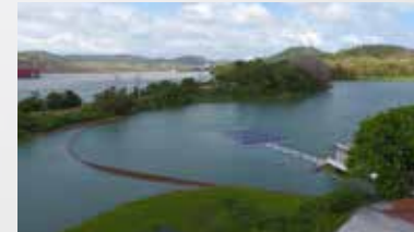
MIRAFLORES, PANAMA - 24 kWp
