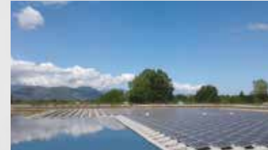
PONTECORVO, ITALY - 343 kWp
